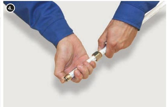
4. Insert the screwed joint body into a pipe till it definitely stops. The joint insertion depth is ca. 9 mm for pipes  $\varnothing 14, 16, 20$  and 12 mm for pipes  $\varnothing 25, 26$ .
