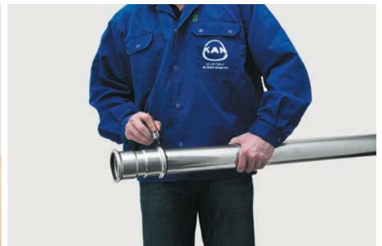
**3 Marking the insertion depth of the pipe in the fitting**
