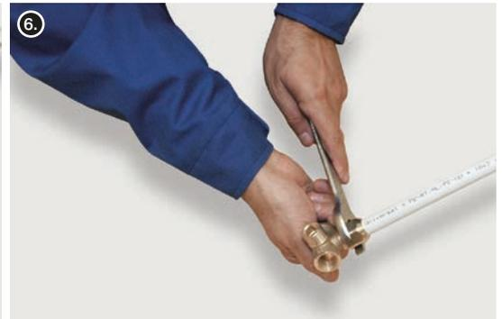
6. Screw the nut onto the fitting body using flat spanner.
